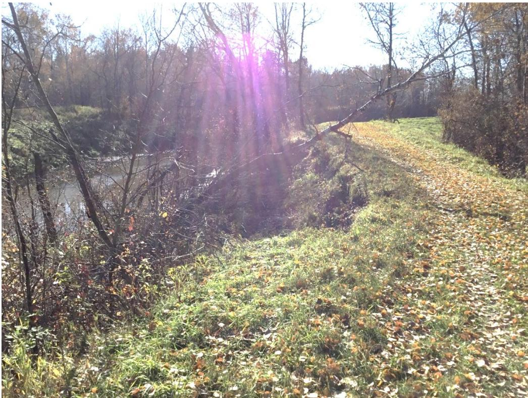
Judicial Ditch 23 outlet stabilization construction was nearly completed, though some touch-up work (slopes were let in rough shape) and buffer planting must still be completed (in the spring or summer of 2022). In addition to the rock structures at the outlet of the ditch, the last 0.6 miles of the ditch were re-sloped and two side water inlets were installed.
